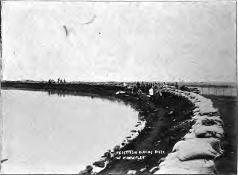
KIMBERLEY—SANDBAGS FORMING A SHELTER FROM WHICH TO REPEL ATTACKS UPON THE RESERVOIR.
